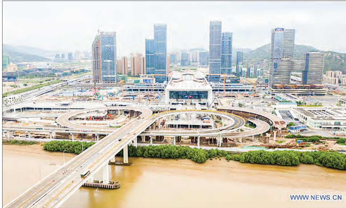
Aerial photo taken on Aug. 18, 2020 shows the Hengqin Port. The new port to facilitate travel between Macao and Zhuhai, south China's Guangdong Province, was officially put into use, a new step to boost development of the Guangdong-Hong Kong-Macao Greater Bay Area. PHOTO: XINHUA/CHEONG KAM KA
