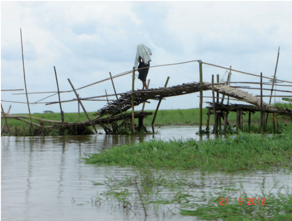
Community-built footbridge replaced the storm-damaged culvert (A. Somesan)
