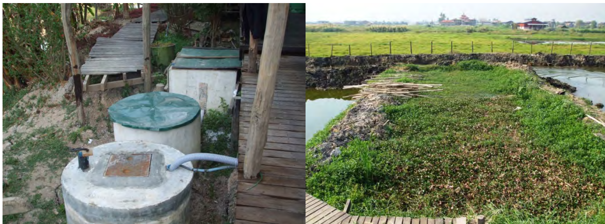
Figure 1 Tertiary treatment system for wastewater at Heritage House in Inn Kyaw Phone village, Inlay Lake, with wetland treatment final stage
