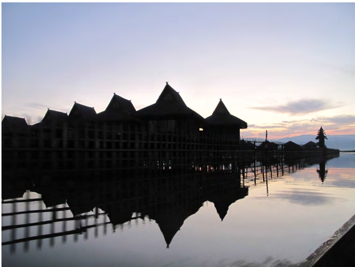
Figure 40 Shwe Inn Thar Hotel, Inlay Lake
