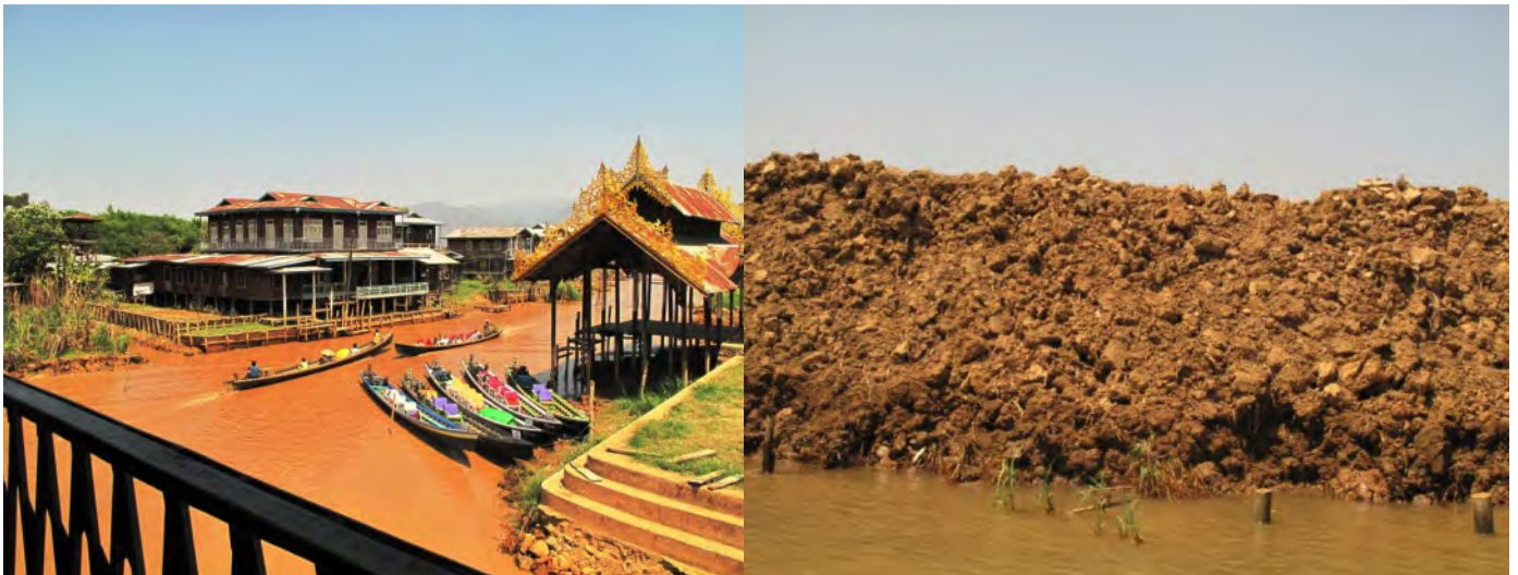
Figure 24 Yellow silt has been washed off unsecured earthen banks by boat traffic around Ywama – it is not coming from the higher catchment
