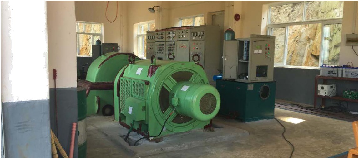
Figure 3.14 Kanbauk Hydroelectric power stati
