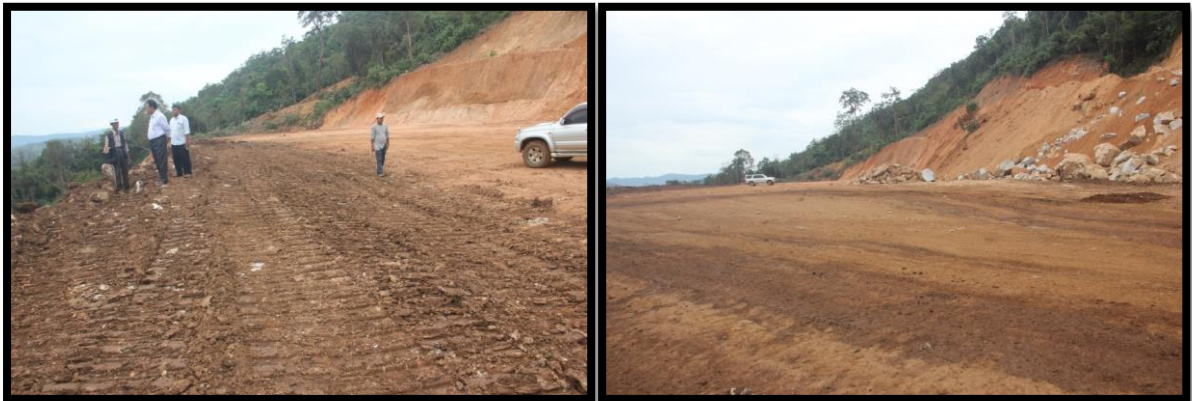
Figure 14.3 Upper part of stock yard site
