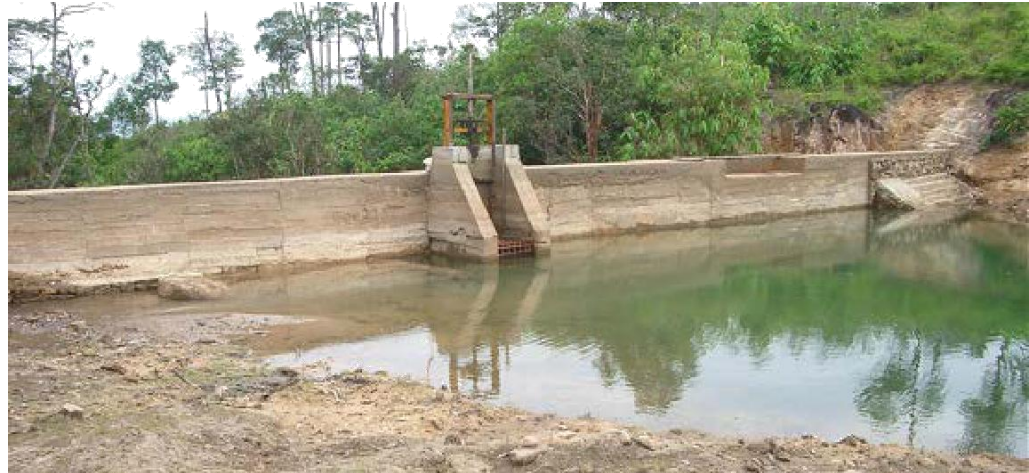
Figure 3.16 Balu Dam (in dry season), showing entry to discharge pipe and spillway
