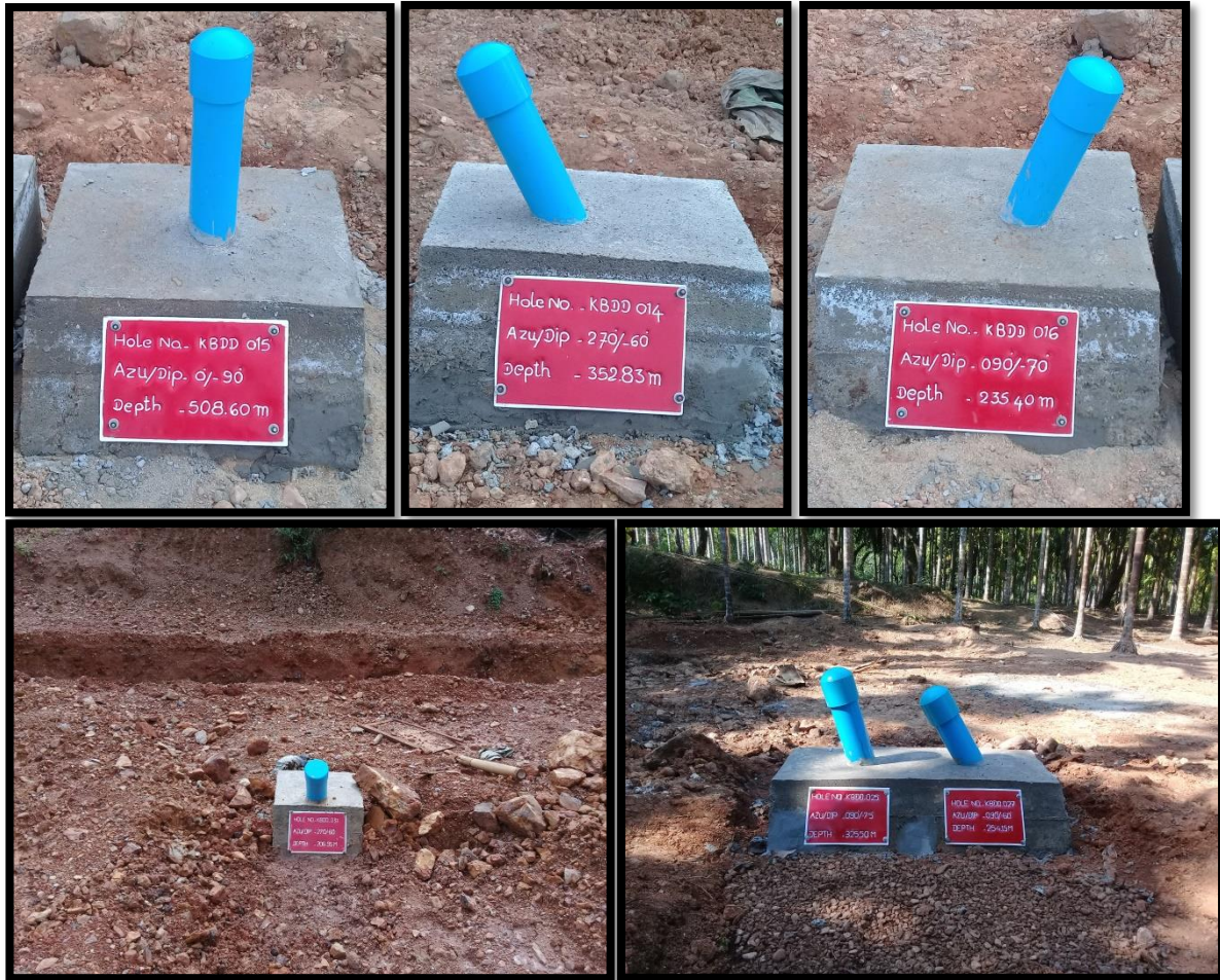
Figure 14.6 Drill hole caps
