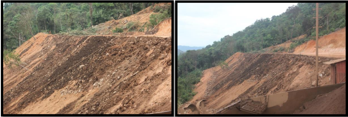
Figure 14.2 Under construction of retaining wall stock yard
