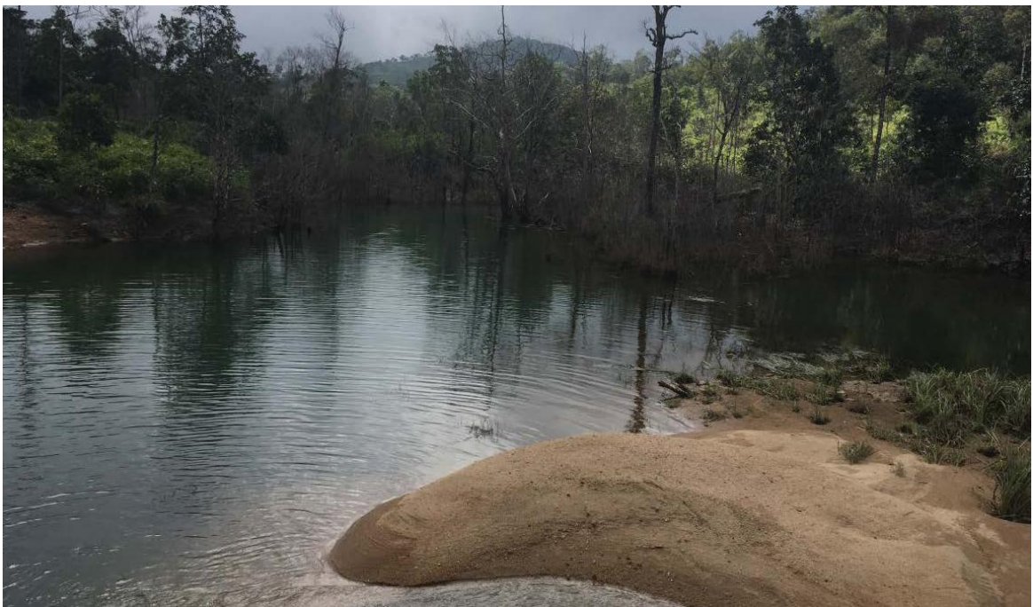
Figure 3.15 Balu Dam in Wet Season
