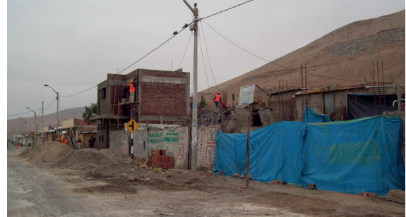
Figure 6. Construction in Ite, Peru
