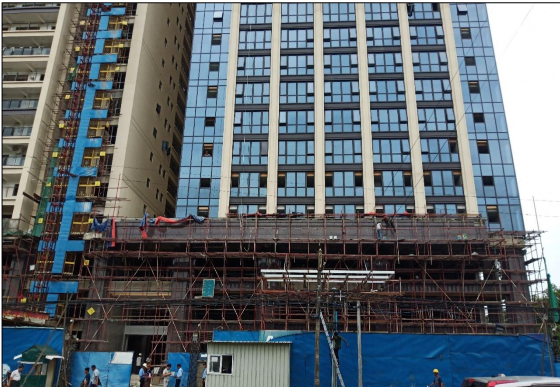
Figure 3-1 Construction Site of the Project
