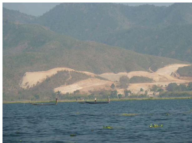
Figure 10: Hotel Zone landscaping works from Inlay Lake
