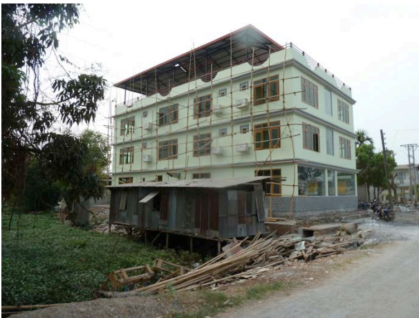
Figure 13: A Hotel under construction in Nyaungshwe
