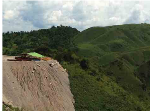
Photo 30: Loose soil pushed over the hill side bordering Bilu stream
