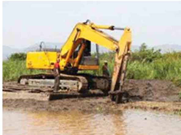
Photo 21: Excavator digging silt and dumping it on the near shore
